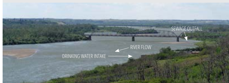
(above) Pathogenic Cryptosporidium from the sewage outfall (in front of the bridge) passed through the drinking water treatment plant at North Battleford, Saskatchewan causing an outbreak of illness affecting an estimated 6000 consumers in March / April 2001.
