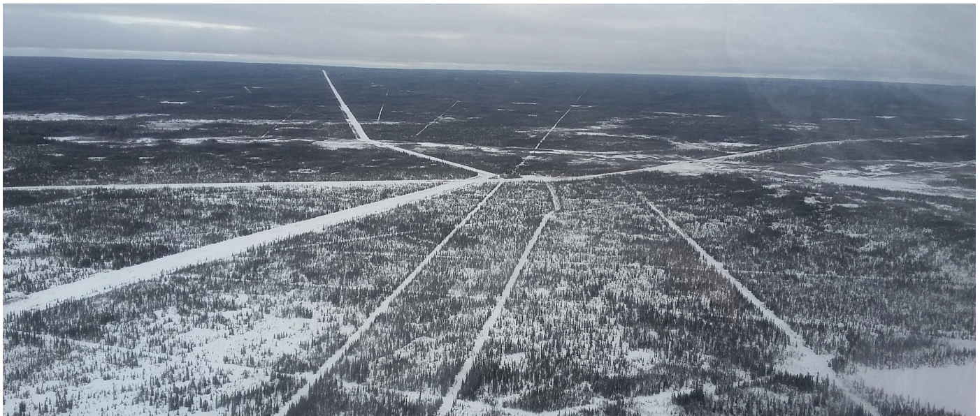
Linear disturbances (seismic lines, pipe lines, roads) in northeastern BC; these features accelerate permafrost thaw and enhance drainage from the landscape.
