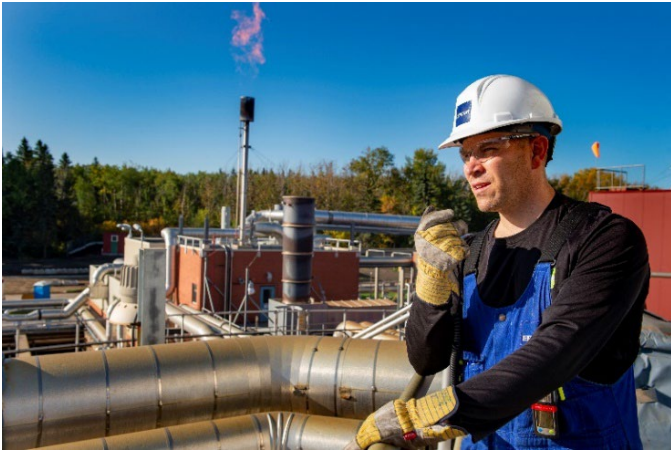
Figure 5: Gold Bar WWTP, with biogas flaring visible.
