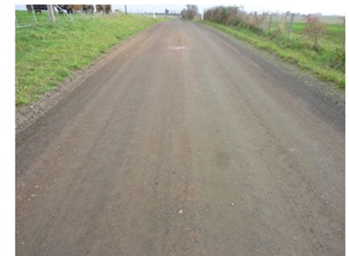
Level of service option 2 Unsealed road Graded 2 times per year Resheeted on 5 year cycle Operating cost $10,000 per year
