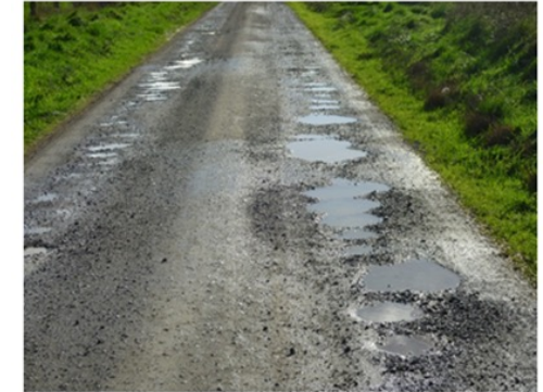
Level of service option 1 Unsealed road Graded on 2 year cycle Resheeted on 20 year cycle Operating cost $2,000 per year
