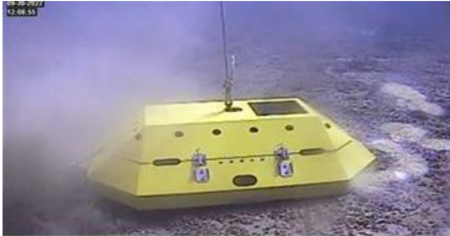
Clark WTP ADCP Installation – Sept 2022
